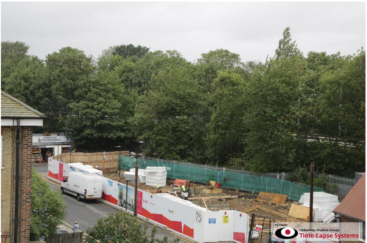
Socially distanced work on site to build Joy Gardner House - eleven new Council homes at Templeton Road, Seven Sisters
