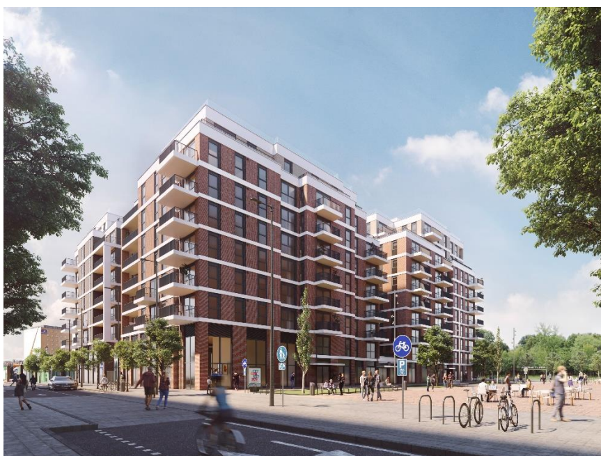
Rosa Luxemburg House, Tottenham Hale – on site with 104 homes completing March 2022
